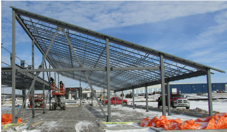
STEEL FRAME STRUCTURE FOR THE OFFICE, DESIGNED BY BRADLEY ENGINEERING.
